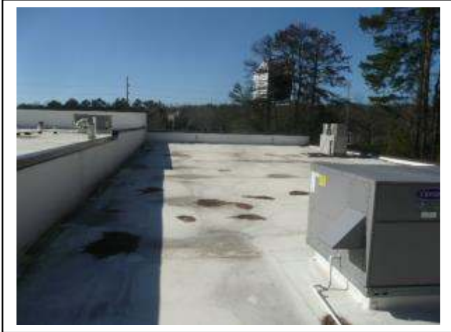
Overview of TPO roof suites 2,3
