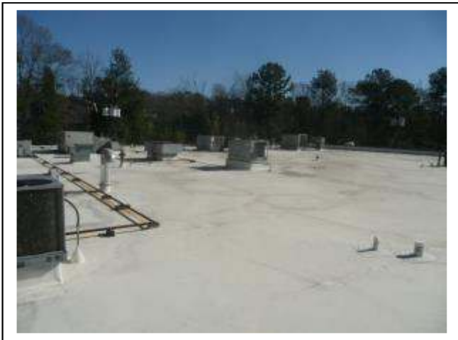
Overview of TPO roof suites 4,7,8
